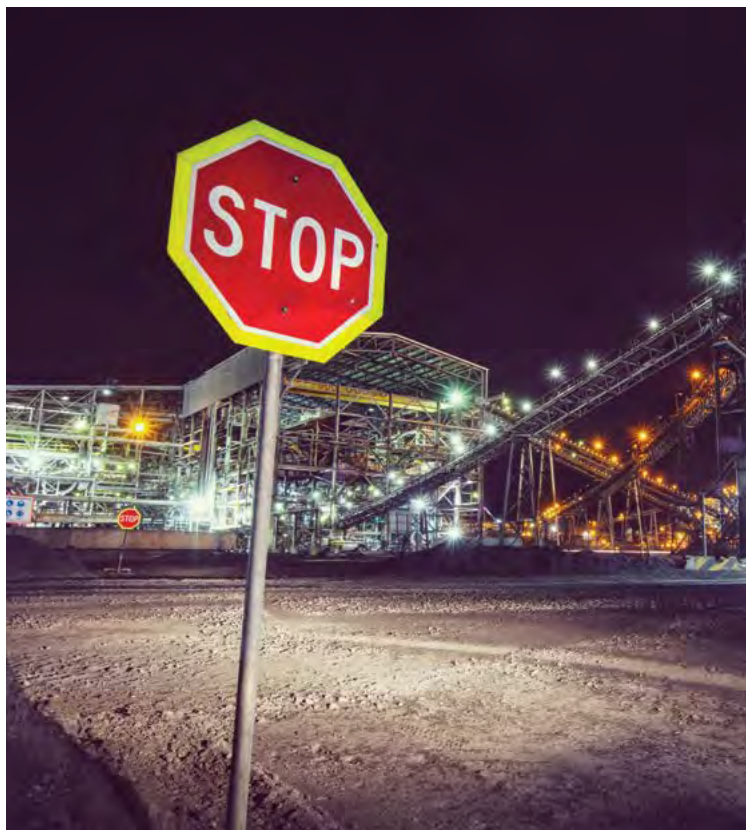
Below Coal Handling Preparation Plant, Curragh Mine
